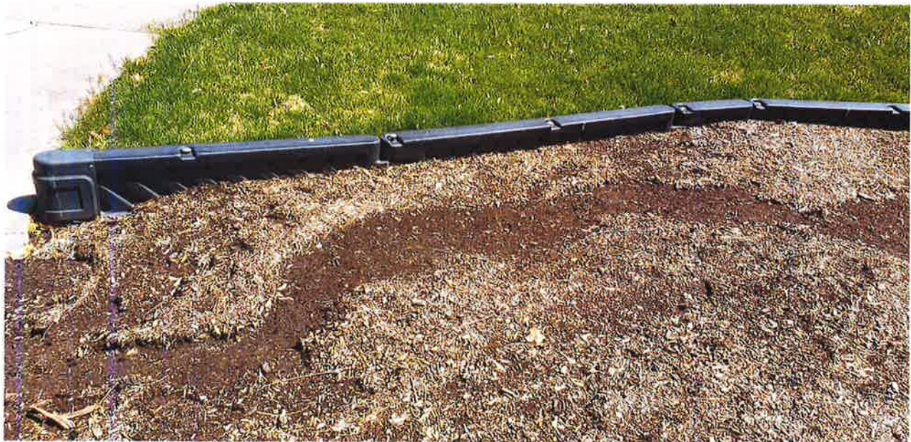
Drainage issues near the entrance to the playground area from the sidewalk. Runoff from the adjacent slope is eroding the Fibar surfacing.
