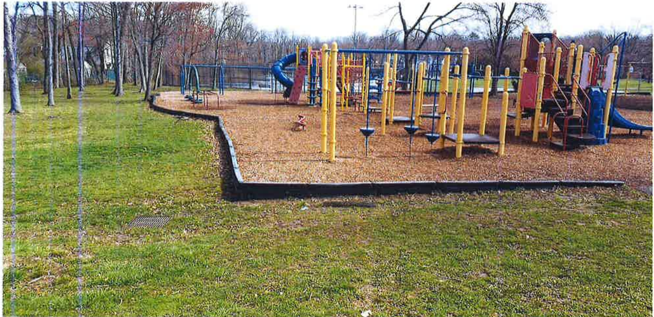
View of the large 5-12 play structure, fading of the red and blue components are visible.
