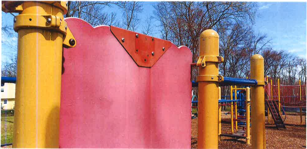
Example image of the fading typical on the playground structure, image also shows some missing hardware on the panel piece.
