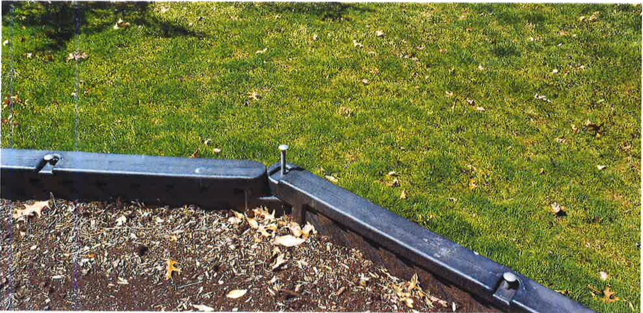
Stakes from the plastic curbing are protruding in several locations and are tripping hazards
