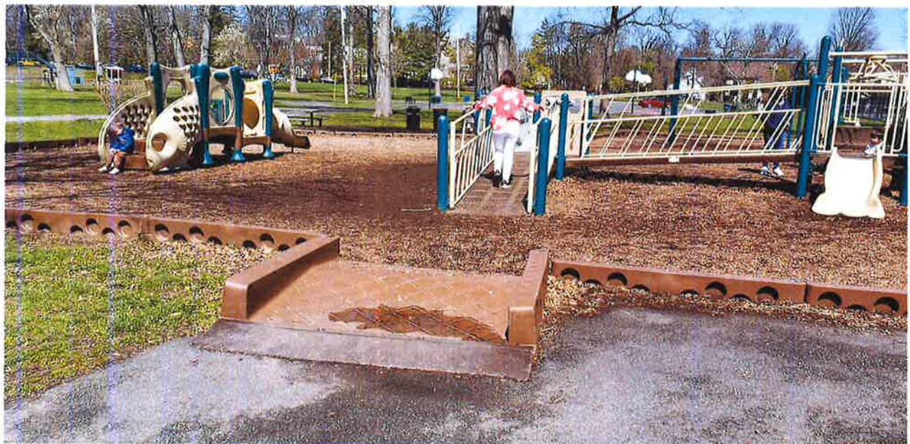
View of the plastic transition piece from the asphalt pavement walkway to the fibar surfacing at the playground entrance located behind the park office building.
