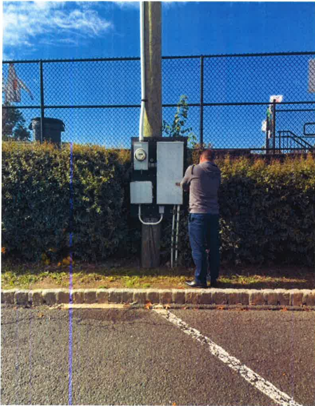
Photo 3 – Upper Tatlock Field Electric Utility Service Meter and Distribution Panel
