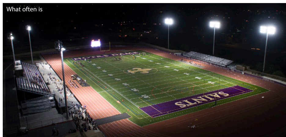
2016 · Other manufacturer's fixture with LED light source after an attempt to resolve glare complaints Notre Dame Preparatory High School, Scottsdale, Arizona, USA
